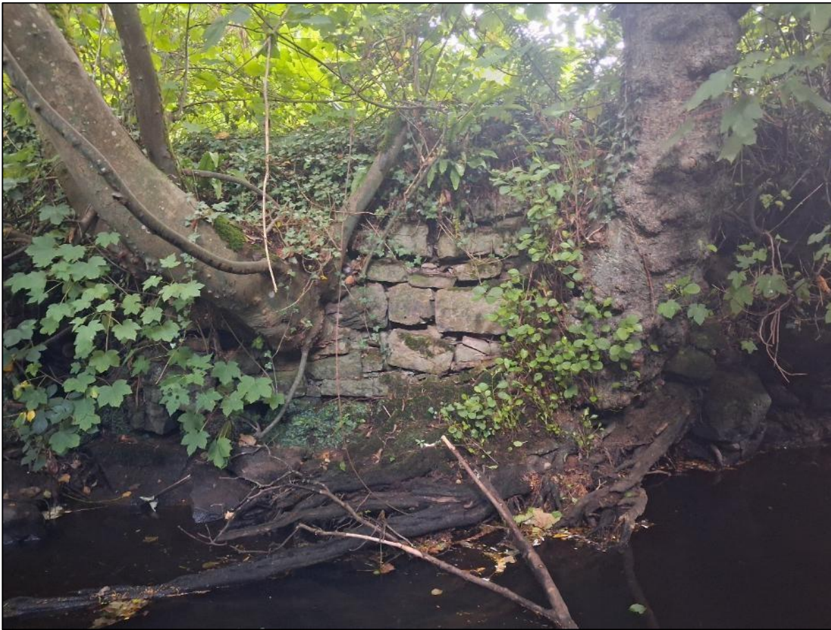
Figure 12 Stone revetments of Small River upstream of proposed footbridge
